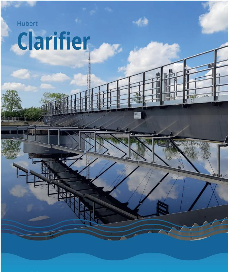
Hubert clarifiers or scraper bridges provide continous low-cost separation and removal of suspended solids from wastewater.
